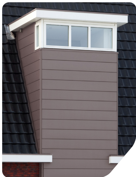
Architect: Meerhuis bv
